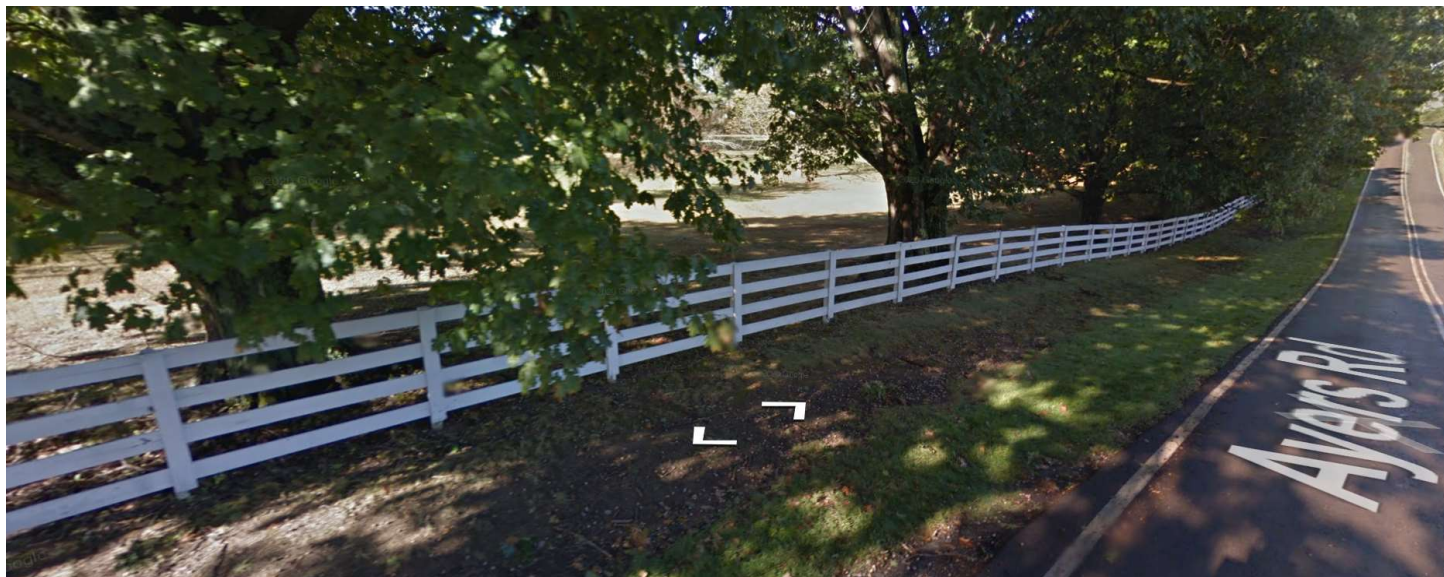
View of site from Ayers Road looking west (Google Streetview)
